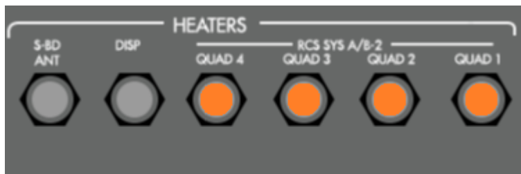
Heater circuit breakers on P16
