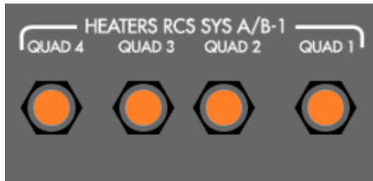
Heater circuit breakers on P11
